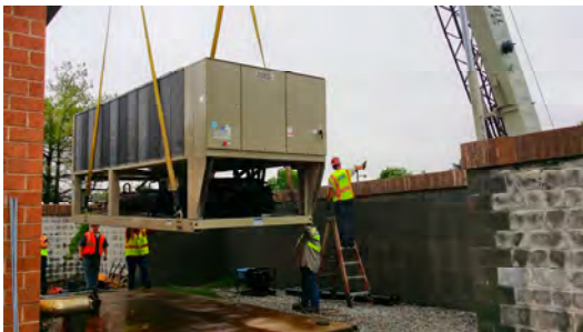
Daikin Chiller Replacement Project Quantico VA
